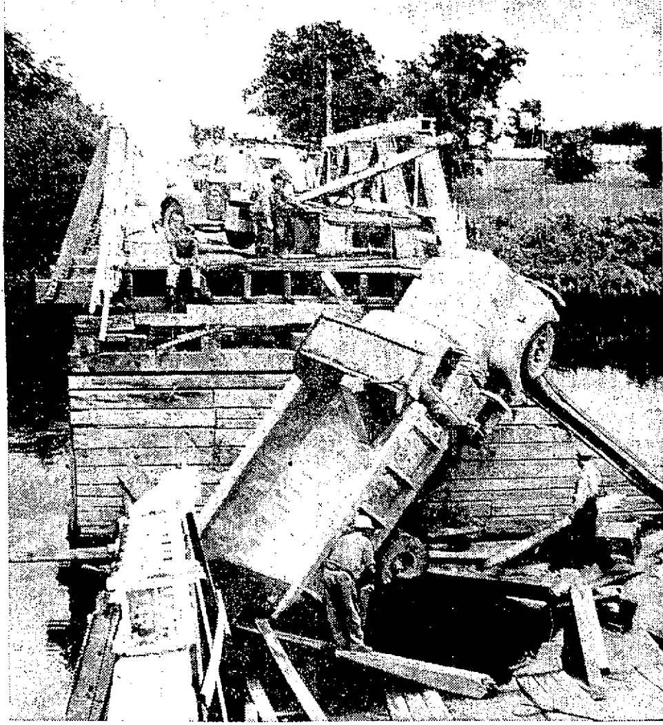
The only damage done when a tandem truck crashed through a bridge over the Whitemouth River in Whitemouth was the loss of a load of gravel and the use of the bridge. Truck driver Sylvester Slynkewich of the town was not injured. Road traffic has been stopped since the accident occurred Wednesday. Police say there were no load restriction signs to warn heavy vehicle operators.
